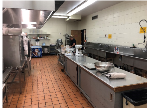
Quarry tile in the kitchen is in good shape.
