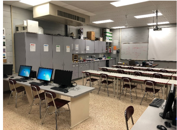
The epoxy flooring in the STEM area is in good condition.
