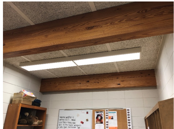
Ceilings on the main level with exposed wood beams.
