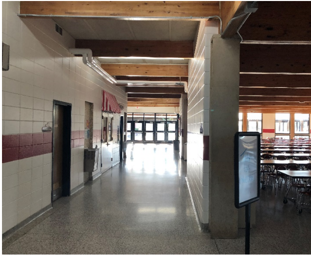
Terrazzo flooring throughout the corridors and cafeteria are in good condition.
